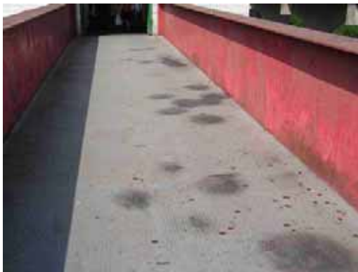
Photo 20: Surface of footbridge from East Lane House.
