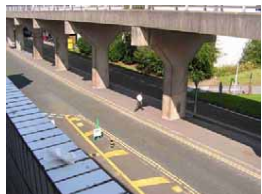
Photo 3: Pedestrian crossing road at ground level
