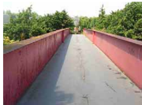
Photo 2: Footbridge towards Asda
