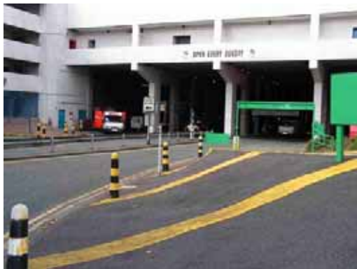
Photo 5: Service roads underneath mall
