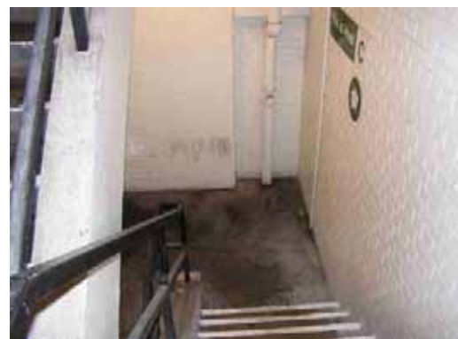
Photo 7: Non-refurbished stairwells at multi storeys
