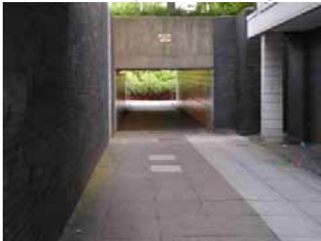
Photo 18: Underpass below Northway
